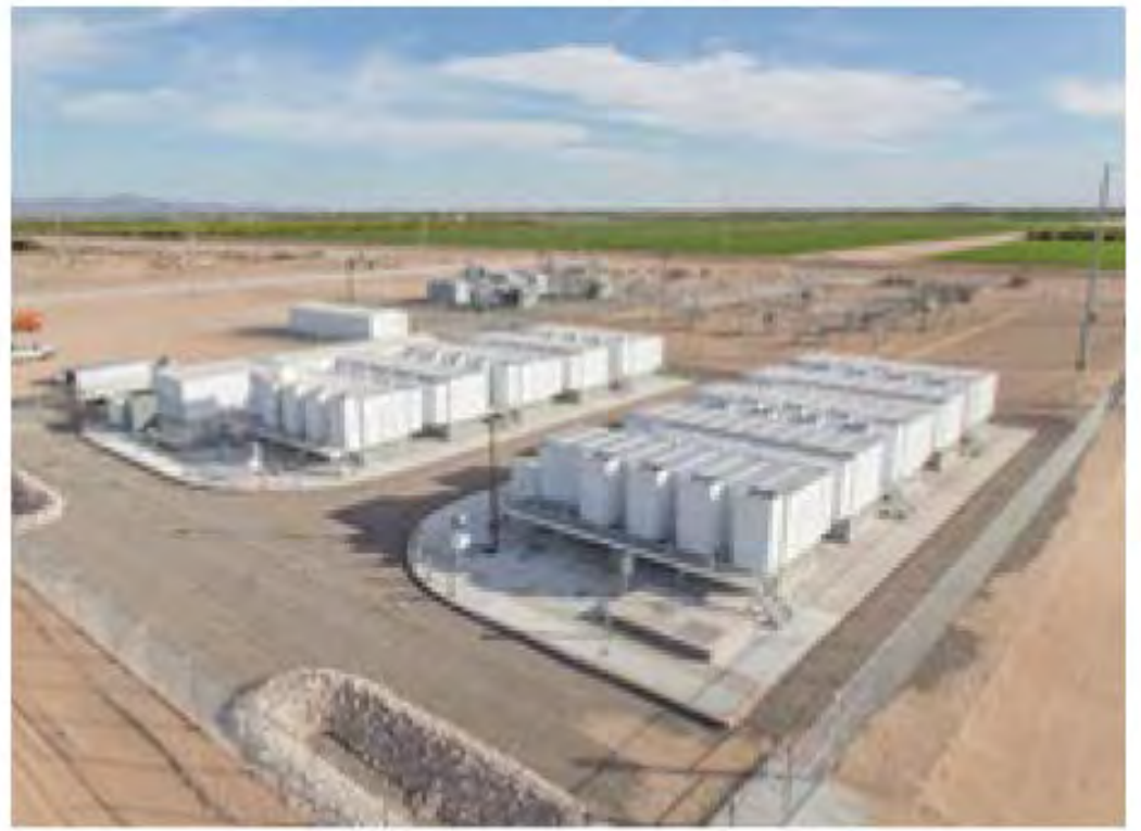
Yuma Microgrid (MCAS)
